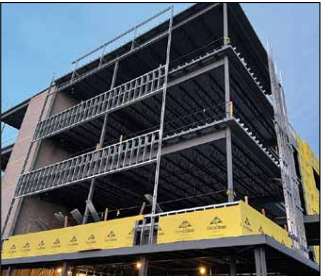
The BOTRI team used metal framing, batt insulation and drywall on the four-story structure.
