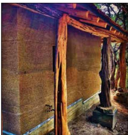
Per Japanese tradition, the beams must be burned and hand-brushed to keep bugs out of the structure.
